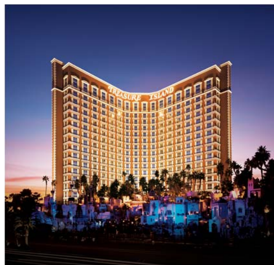
Treasure Island Hotel Size: 36 floors, 2885 rooms Built: 1993
